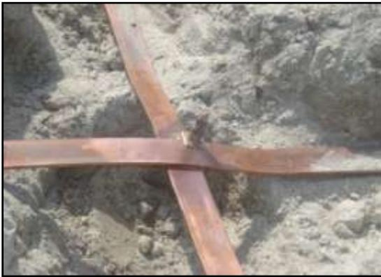
Fig.3 - Overlap joint between conductors at 90 degree [2]
